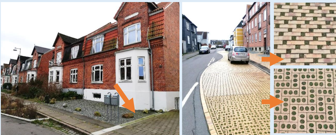
Figure 19: Skibhus: The decoupling of rainwater by citizens, the arrow indicating where rainwater is decoupled and led to the retention on the public road (left) and the experimentation with street profiles (right) (Author, 2020).
