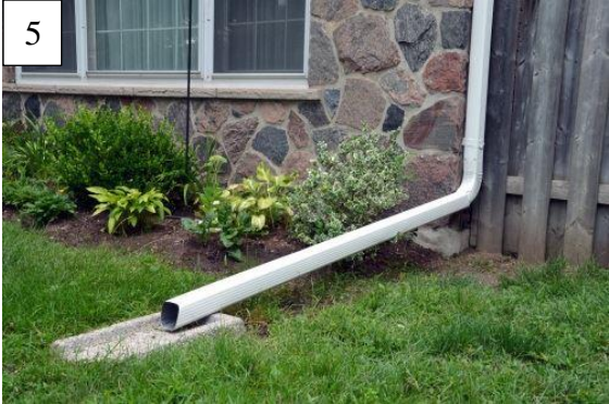
Figure 10. Disconnection of downspouts
