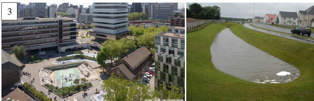
Figure 8. Dry detention basins
