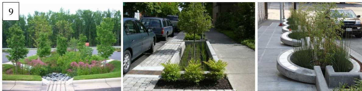
Figure 14. Rain gardens, rain beds and planter boxes
