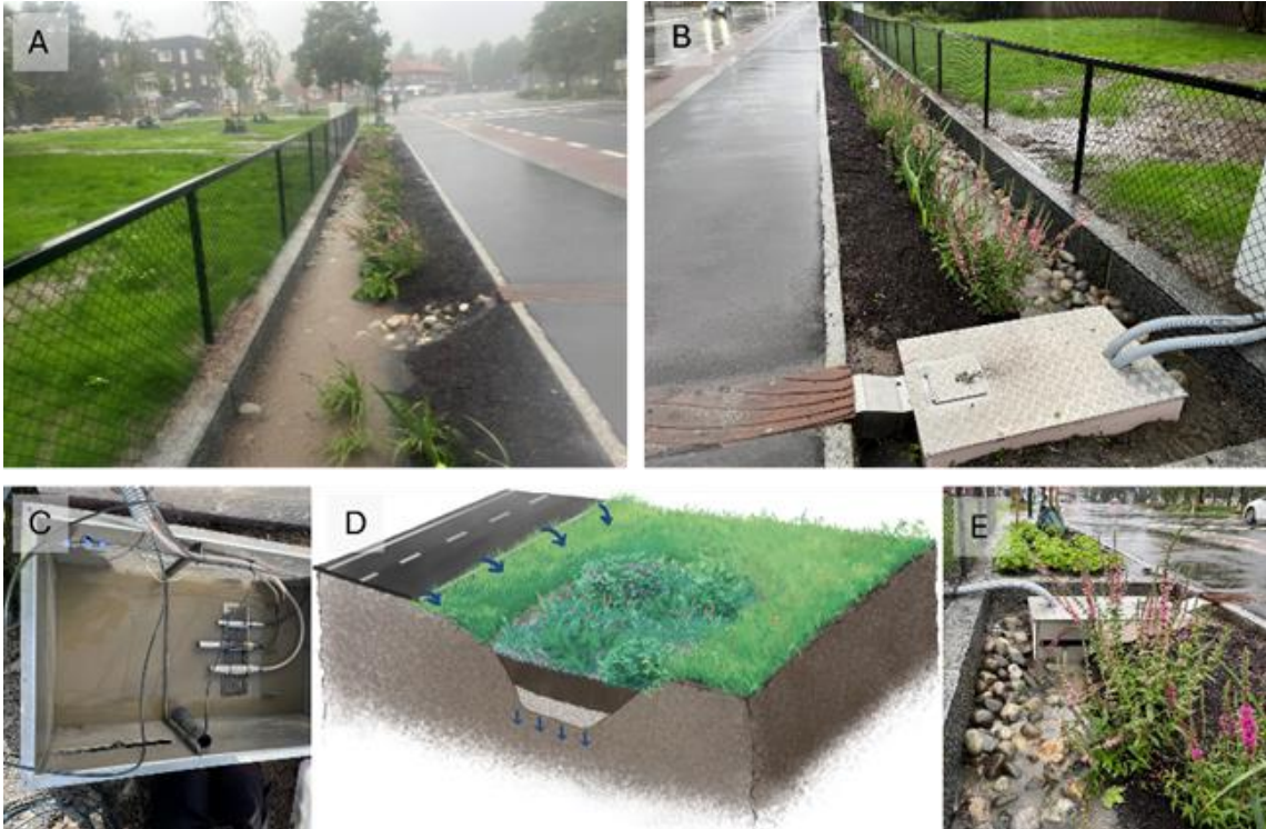
A) Heavy rain event (August 2023), B) the influent monitoring box, C) sensors installed in the influent monitoring box, D) illustration of raingarden with treatment from road runoff, E) the raingarden and the influent monitoring box showing water flowing over the v-notch.
